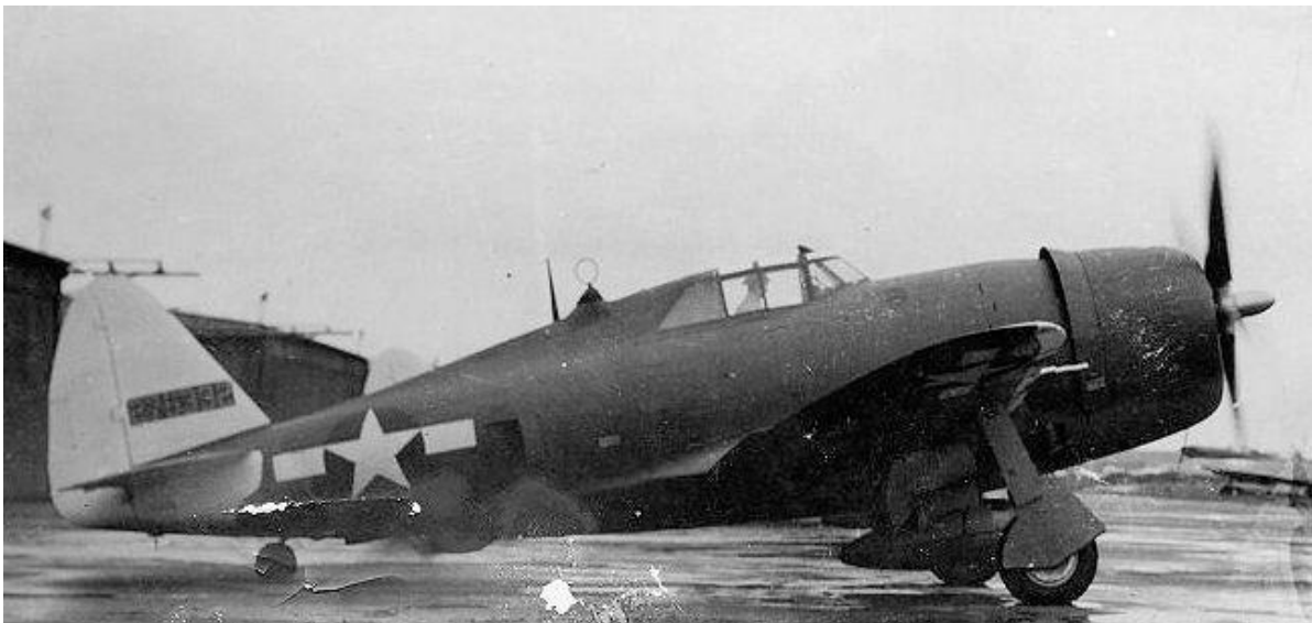
P-47D-11-RE 42-75332, "somewhere in Australia", which later served in 311th Fighter Sqn, 348th Fighter Group, then marked as V69. Note DF Loop Antenna.
